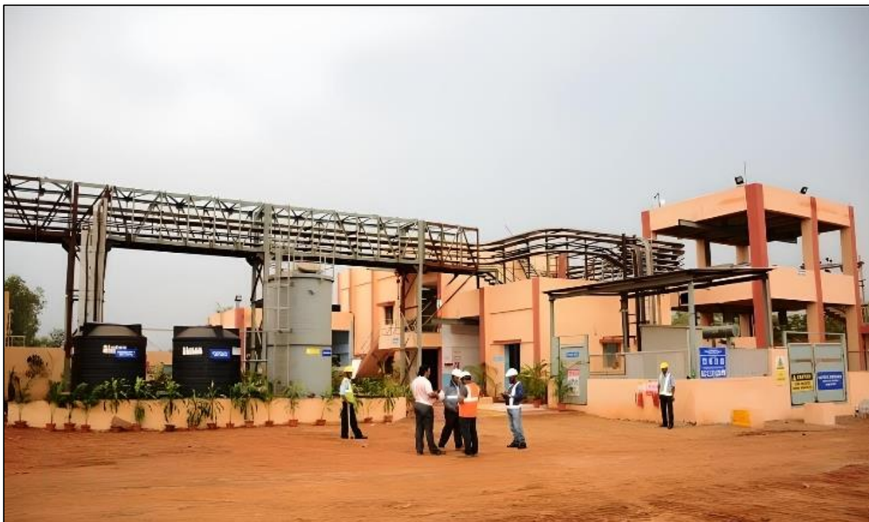
Acid dyke area with safety Arrangements
