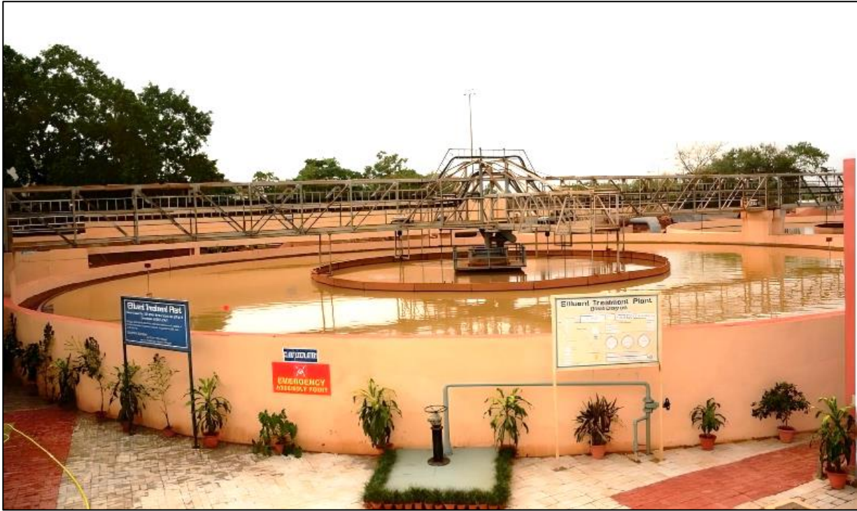
Chromite Mine Effluent Treatment Plant
